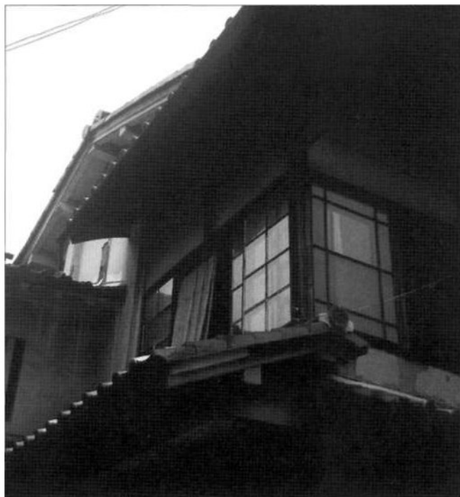
The upstairs window of Nijo jinya in Kyoto. The glazing is a modern addition.
